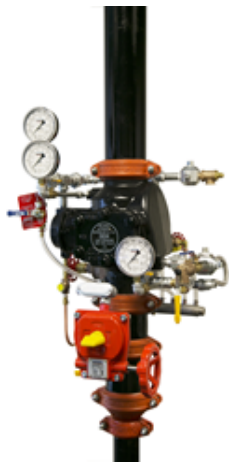
DDX-LP Dry Pipe Valve System
